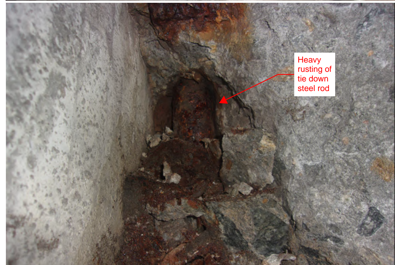
Cantilever E South Face
